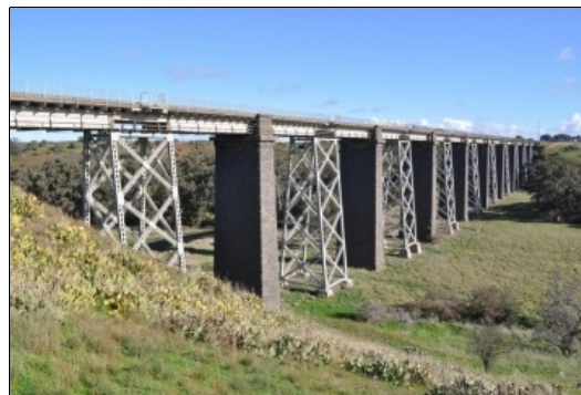
Moorabool Viaduct on Geelong to Ballarat Railway. Peake
