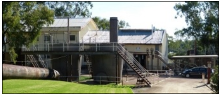
Water towers & discharge pipe of the Humphrey Pump at Cobdogla
