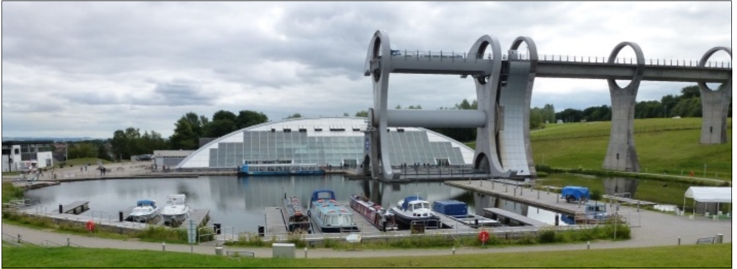
The Falkirk Wheel Basin, Visitors' Centre (rear), entry aqueduct from the Forth & Clyde Canal (right), and the Wheel itself (centre right). View from West. K.Baker
