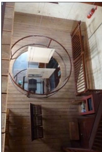
Upper Level of the Burra Engine House
