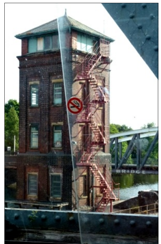
Control Tower, Barton Swing Aqueduct.
