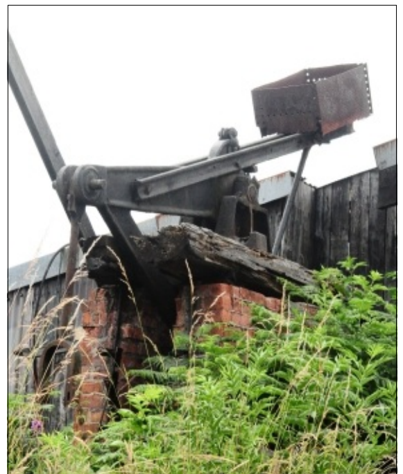
Beam pump at Lion Salt Works
