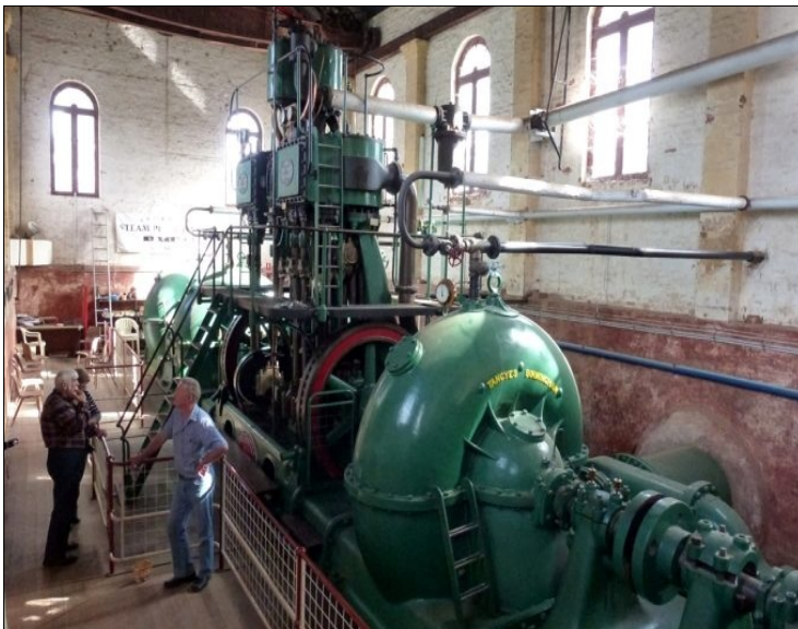
The Chaffey designed vertical triple expansion pump engine on the Murray River at Psyche Bend near Mildura, Victoria. Photo Keith Baker
