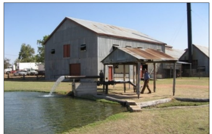
Artesian bore, woolscour (rear) & powerhouse (right) Photo B.McGrath
