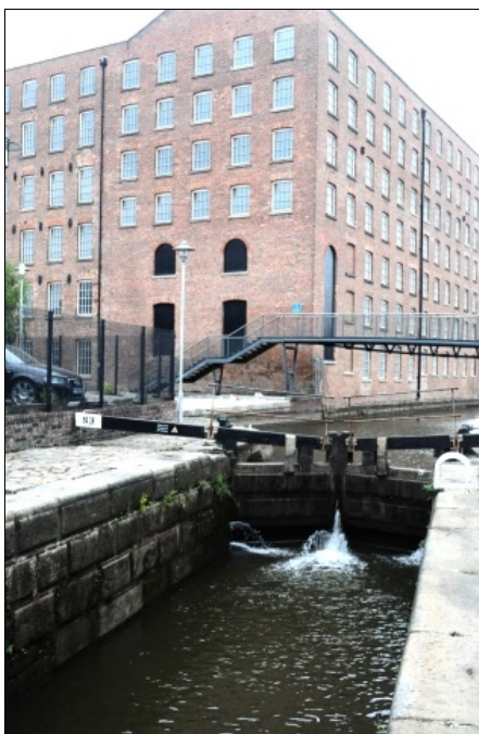
Warehouse & canal lock at Ancoats O.Peake
