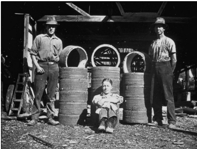
D.J. Byles, Jack Brown & F. Shinn with a stack of finished pipe collars.
