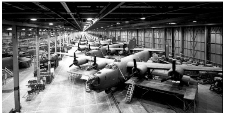
B-24 Liberators under construction at the Consolidated Factory at Willow Run, Michigan USA Image: US Army Signal Corps, 1940 to 1945.
