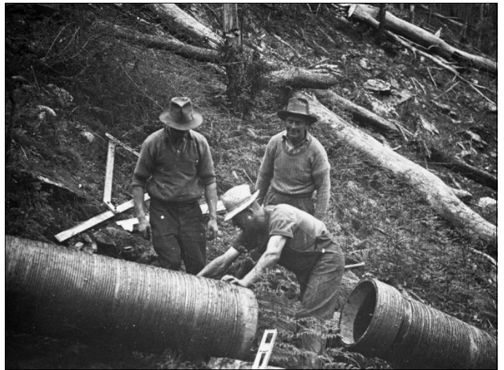
J. Hearn, George C. Brown & Mick Waters putting the pipeline together.
