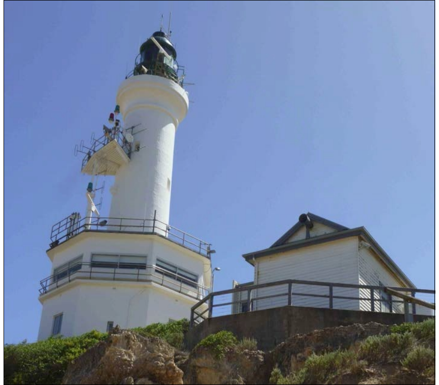
The foghorn shed next to the Point Lonsdale Lighthouse.
