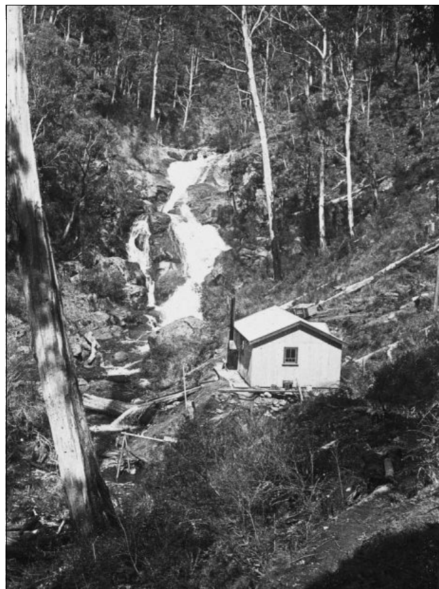
Gilmore Falls Powerhouse c1934.
