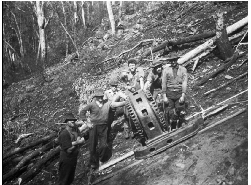
"How the Machinery Went Down" – sliding part of the Westinghouse alternator down the hill. Note the heavy rope, the man with a crowbar and the family dog taking an exciting ride.
