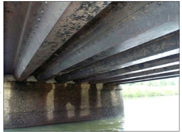
Soffit of the bridge deck
