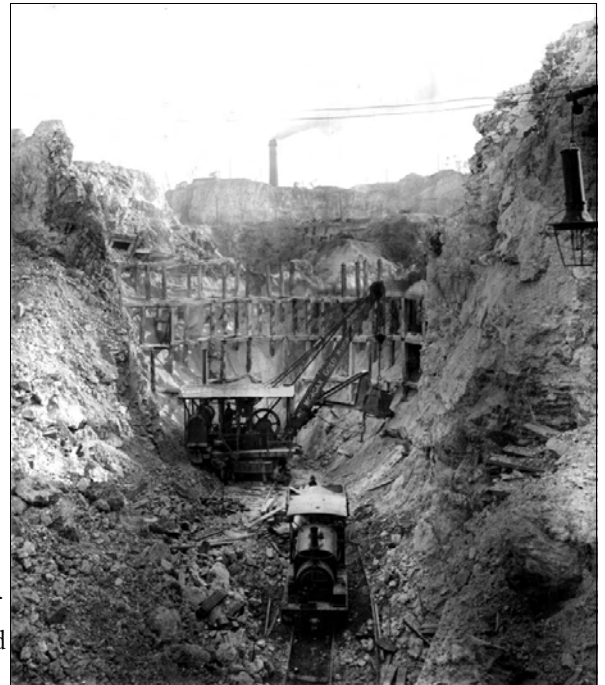
Image below: Whitaker excavator and Hunslett locomotive working in a difficult position mining out the old stopes, circa 1908. The Copper Works stack is in the background.
