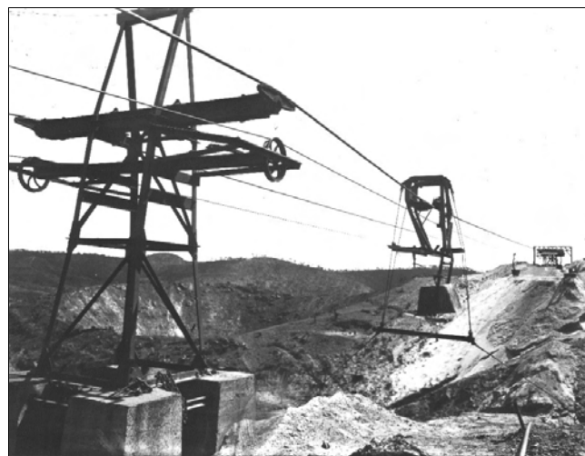
Image above: The aerial tramway or cableway at the mountain top showing the headworks. CAPCOL Collection.
