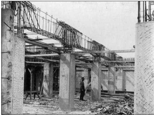
Left: Central Station North Concourse under construction with some of the roof reinforcing in place. 18-11-1924. ARHS NSW - RRC5174919
