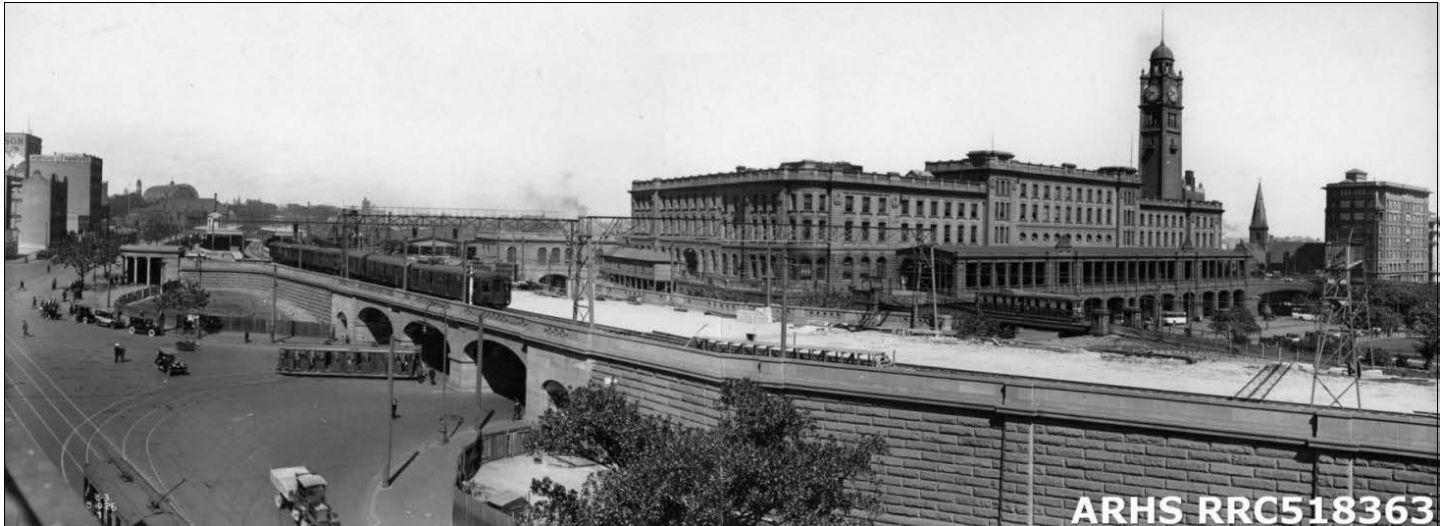
A circa 1926 composite photo of the Eddy Avenue Bridge which appeared in John Bradfield's paper on "The City Railway" in the IEAust Transactions of 1926. Taken from the roof of a building in Elizabeth St, looking south-east. It shows, left to right: the grand Chalmers St entrance to the new electric train stations at Central; the three spans of the Eddy Ave bridge with an electric train standing on the bridge and a tram exiting from under the central span; the 1906 Central Station building, clock tower and colonnade; a tram entering (or leaving?) the Colonnade over the Eddy Ave tram bridge; the spire of Christ Church St Lawrence; and Daking House, far right. Image: Australian Railway Historical Society, NSW, Railway Resource Centre (ARHS NSW - RRC518363).
