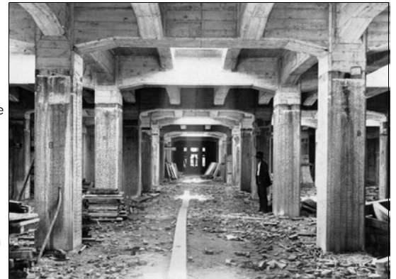
Left: Central Station North Concourse under construction with some of the roof reinforcing in place. 18-11-1924. ARHS NSW - RRC5174919
