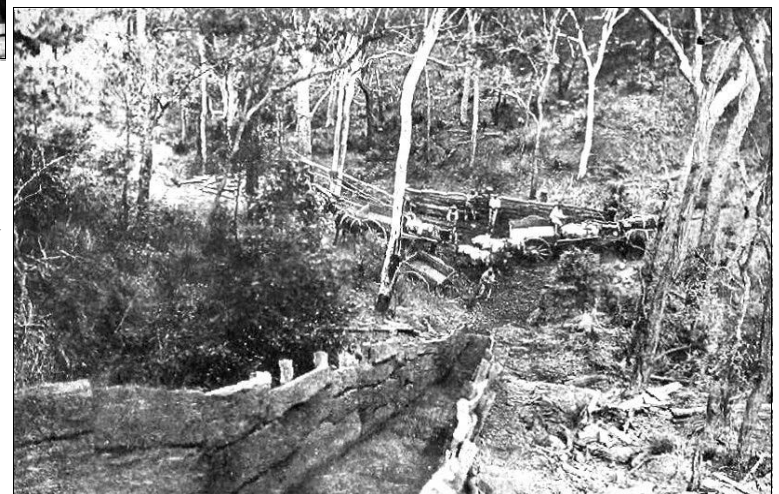
The 'shoot' [Morgan's spelling] passing ore from the top quarry to drays for transport down the mountain to the riverside stamp battery. The building of this shoot was one of the conditions specified in Morgan's letter to Hall. Image: CAPCOL Collection.
