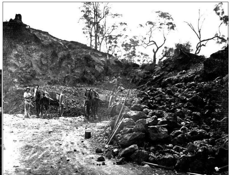
Loading ore into drays in the top quarry. Wesley Hall, the Mine Manager from 1882 to 1891, said "Six men can comfortably break sufficient stone to keep the battery supplied". Image: Hempseed Collection.
