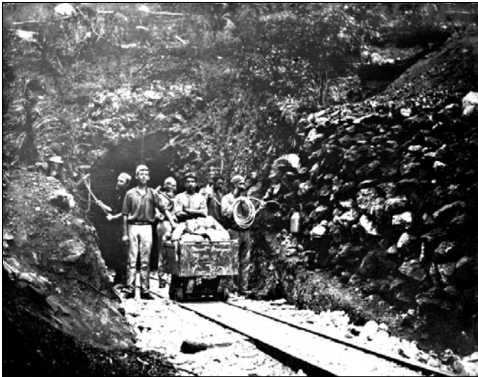
When mining was extended to include underground tunnels, ore was pushed out by hand in little rail trucks but still dumped into drays for transport down the hill. Image: CAPCOL Collection.
