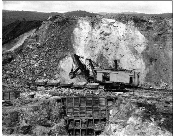
Image above: The Bucyrus excavator removing the remnants of the oxidised gold ore, old stopes, sulphide ore and waste, circa 1905.
