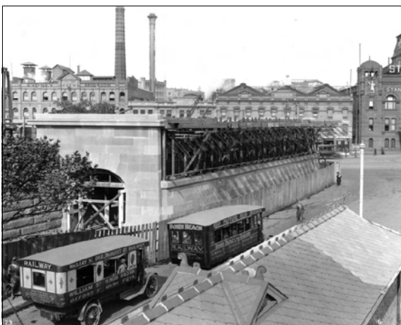
Left: The North footpath span completed. Photo taken 11 Oct 1923.
