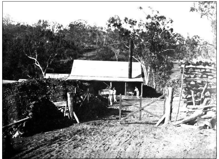
The first stamp battery ca 1883. Note the stacks of firewood, fuel for the battery boiler. Image: Hempseed Collection.
