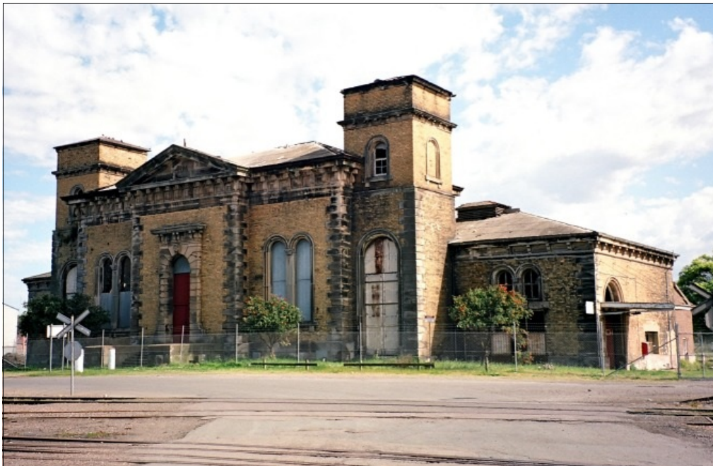
The Hydraulic Pumping Station seen again in 1996, when it was fenced, but still neglected.
