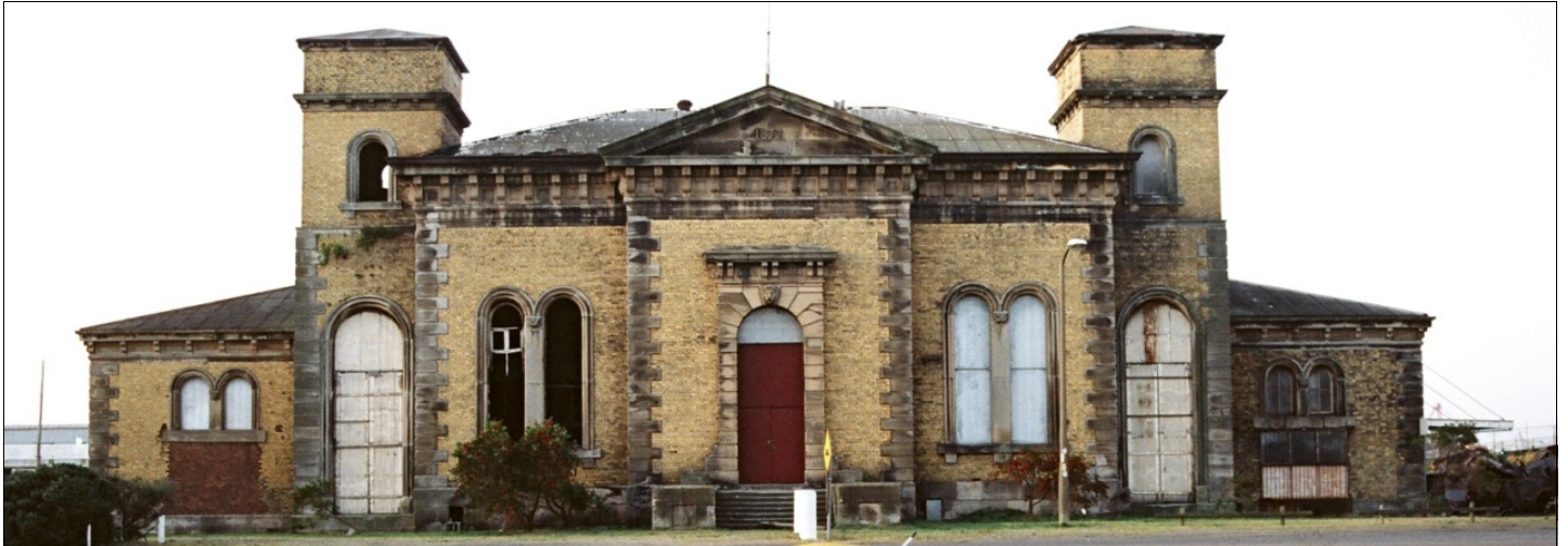
The south, (principal), elevation of the Carrington Hydraulic Pumping Station in 1991, suffering neglect & vandalism.
