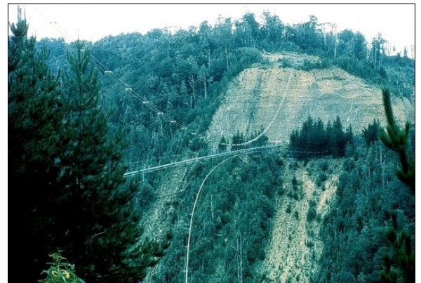
Slurry Pipeline Suspension Bridge, Savage River, Tasmania. Photo from Highest Bridges.com website.
