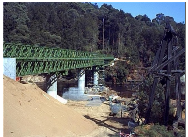
The new Quartermile Bridge.
