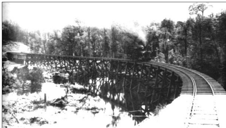
The original Quartermile timber trestle bridge on the King River c1896. Note the double rail on the inside of the curve. Source - Tasmanian Archives Office
