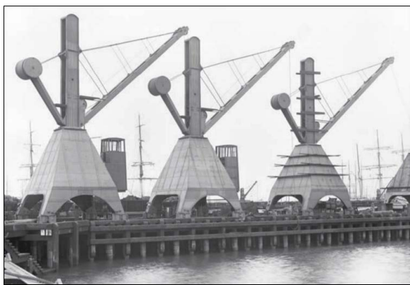
Walking cranes under construction at The Basin east wharf in circa 1901. Photo – Newcastle Library.
