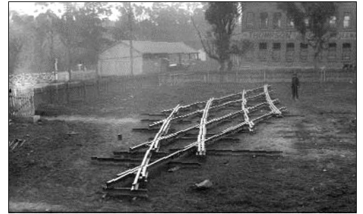
Thompsons built railway points & crossings. This set of two roads crossing two roads was made in 1921 and laid out opposite the factory. Photo Thompsons Archive
