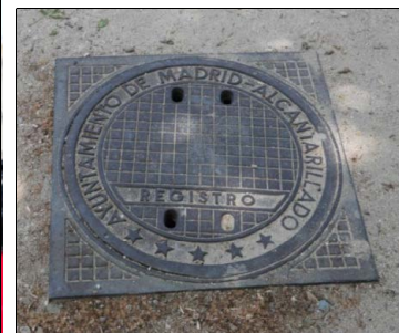
Sewer Cover at Left
