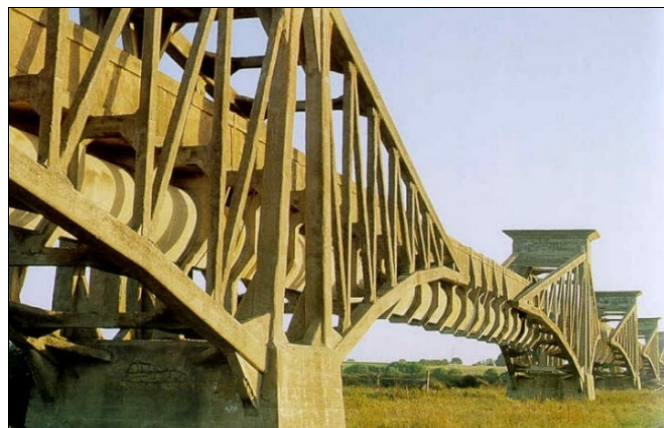
E.G. Stone's Barwon River Sewer Aqueduct at Geelong. Photo – Heritage Victoria.
