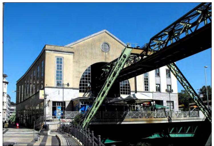
The Kobo Building that replaced the original Doeppersberg station in 1927. From Wikimedia. Photo: Geolina 163, 8 September 2012.
