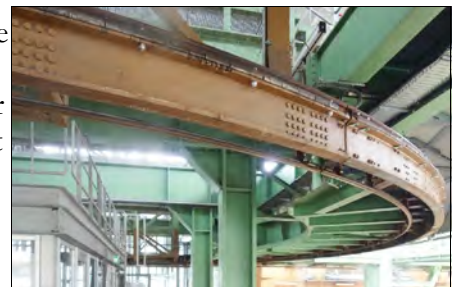
The structure of the Vohwinkel turning loop, clearly showing the live rail inside the loop. From Wikimedia. Photo: Mabit1, 2 August 2020.
