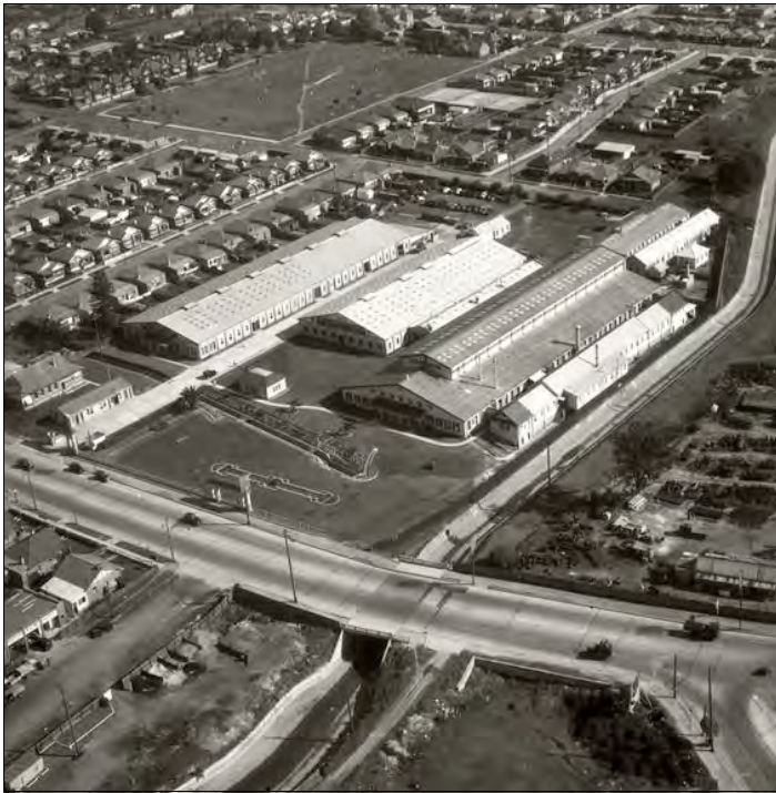
The AWA factory in Ashfield.
