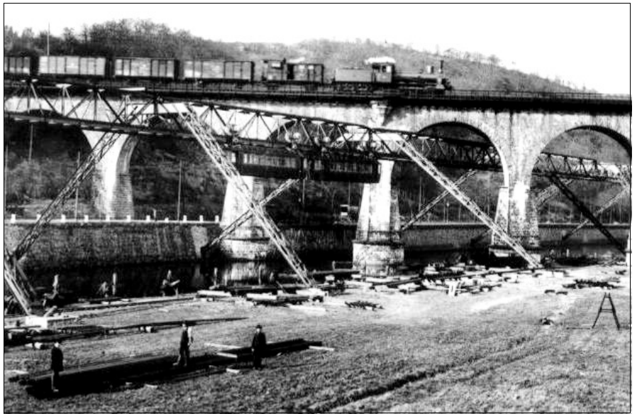
Construction of the Schwebebahn at the Sonnborner Eisenbahnbrücke in 1900. Image: from the Schwebebahn history website.
