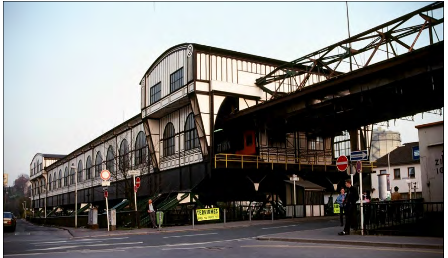
The Oberbarmen car depot, at the east end of the Schwebebahn line. This was a maintenance workshop and held the rail loop where the trains turned back to Vohwinkel. The Oberbarmen passenger station is to the right, out of the picture. Photo: MJ Doring, 1992.
