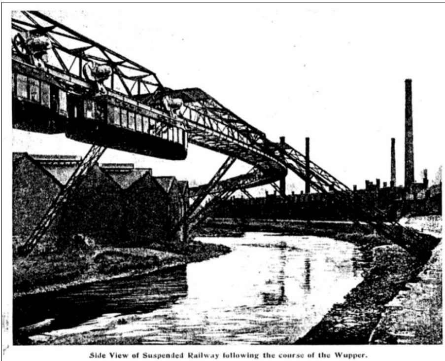
Side View of Suspended Railway following the course of the Wupper.
